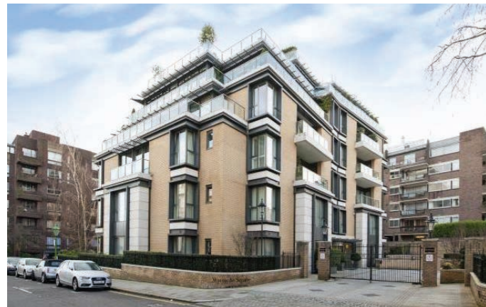
WYCOMBE SQUARE, KENSINGTON W8
